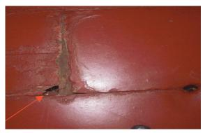
Photo 6: Rotten Floor Boards
