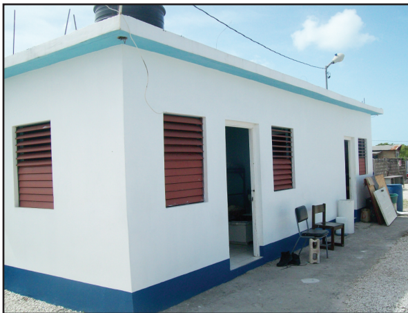
Photo 5: A view of the former kitchen now being used as a Marine Post at the Old Harbour Bay Station.
