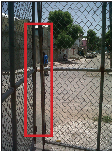
Photo 1: Gate detached from hinges at the Trench Town Station as seen on 28/6/2012.
