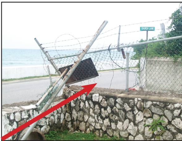
Photo 1: A damaged section of the perimeter fencing at the Sandy Bay Station as seen on 7/8/ 2012.
