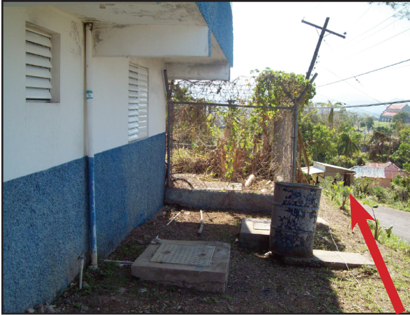
Photo 1: The rear view of the Islington Station showing the absence of perimeter security fencing as presented on 29/10/2012.
