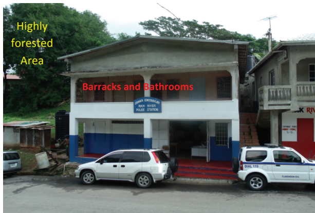
No stairs access from inside Station to barracks and bathrooms as seen on 27/11/12.
