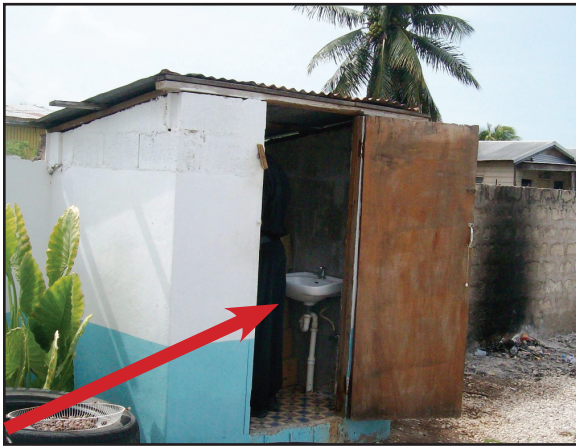
Photo 7: View of outside toilet facilities used by personnel.
