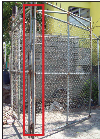
Photo 2: Repaired gate at the Trench Town Station as seen on 21/2/2013.
