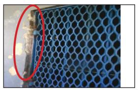
Concrete around the hinges of the cell doors was compromised at the Frome Station in 2018
