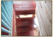
Missing rails and step boards at Mocho Station in 2017
