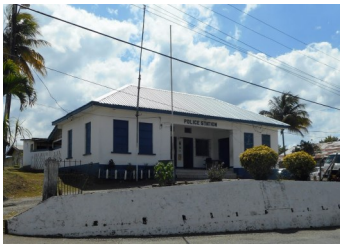
Guys Hill Station in St. Catherine North Division.
