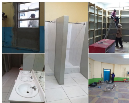
Improvements undertaken at City Centre Station in the Kingston Central Division.
